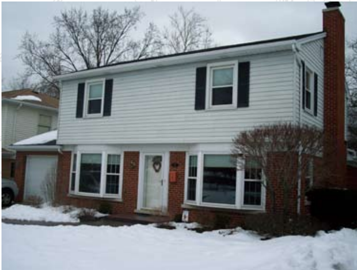
BEFORE EXTERIOR ELEVATIONS
