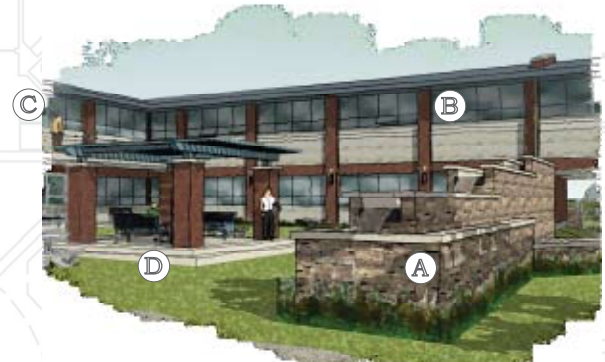
BUILDING IV COURTYARD
